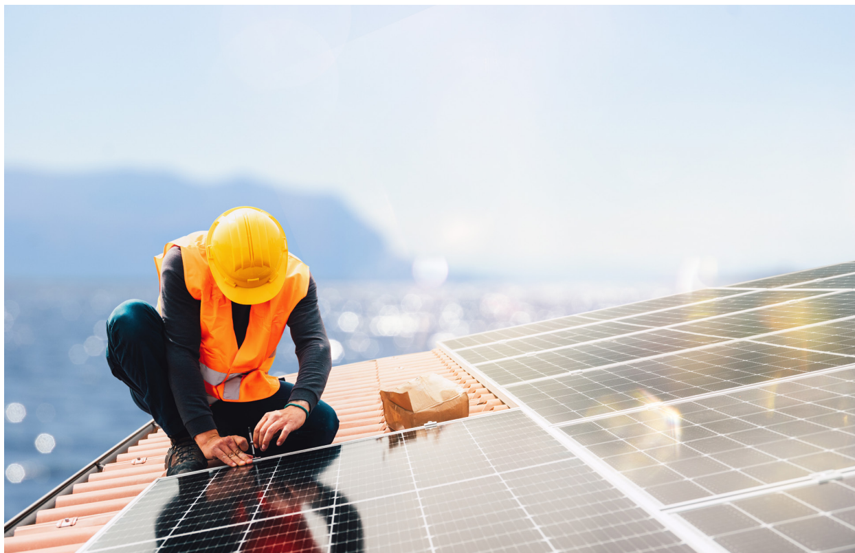
Solar panel installation in progress. (Adobe Stock)
